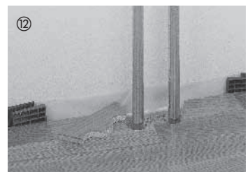
If radiator pipes protrude from the floor, drill and saw a cutout into the board (the size of the cutout depends on the radiator pipe and the required expansion space).
