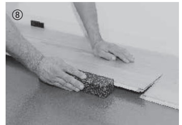
Tap edge gently with tapping block, if necessary.
