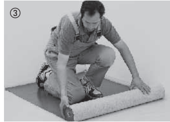
For sound insulation and to smooth out slight irregularities of the subfloor, unroll 2 mm thick luxury insulation layer. Our range of accessories also offers suitable insulation underlays. Asphalt-bitumen felt is not suitable for sound insulation. Parquet with integrated insulation layer is not suitable for glue-down installation.
