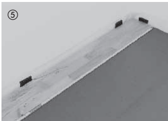
Starting in the right-hand corner of the room, align the boards of the first row with the tongue side parallel to the wall, and fix them in place with wall spacers or plastic spacers as you proceed (always keep an expansion gap of 10 - 15 mm (3/8" - 1/2") around perimeter).
