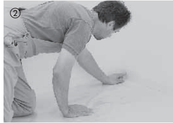
Always use 0.2 mm thick PE film overlapped by 30 cm as an underlay when laying your floor over floor screed. This should overlap in the 30 cm impact area. Extend underlay up all walls. After having installed the skirtings cut underlay at the upper edge of the skirtings.
