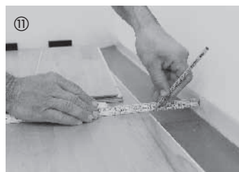
Cut to size and fit in the boards of the last row. Leave a gap of 10 to 15 mm between the boards and wall.
