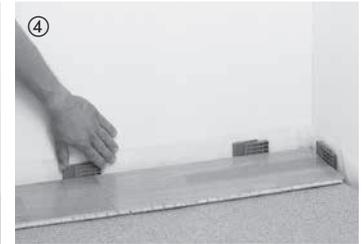
Align the boards of the first row with the groove side parallel to the wall, apply glue to the short sides (see fig. 5) and join the boards together. Fix them in place with spacers, leaving a gap of 10 to 15 mm between the floor and wall. Start the second row with the leftover piece of the first row. This considerably reduces waste (approx. 1% for longstrip).
