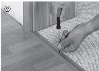
In doorways, mount a suitable moulding system to ensure the necessary expansion space. This also applies if the same floor is to be laid in the adjoining room. In this case, a transition moulding should be used for covering the required expansion gap. Leave an expansion space of approx. 5 mm between the board and the base of the moulding. As a rule, a fine saw must be used to cut a gap the thickness of a board in wooden door frames to allow the parquet to expand.
