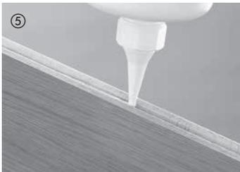
Install the remaining rows by gluing the tongue-and-groove joints on the long and short sides. Apply glue along the entire length of the top side of the groove.
