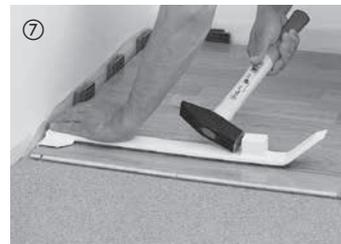
Use the pull tool to join the last board of the row onto the previous board. Set distance spacers. Proceed in this way row by row. The pull tool can also be used for fitting boards under radiators.
