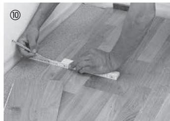
When you reach the last row, trace the distance from the wall on the boards for this row. Leave enough space for an expansion gap of 10 to 15 mm between the boards and the wall. Cut the boards to size, apply glue and join them with the pull tool.
