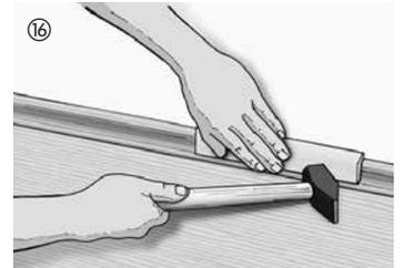
After installation the distance spacers are removed and the skirtings (with or without clip system) are fastened to the walls – that's it.
