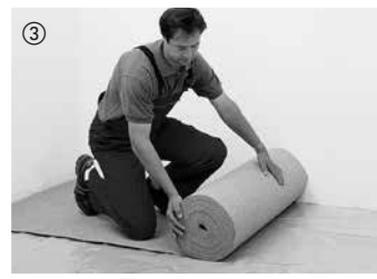
For sound insulation and to smooth out slight irregularities of the subfloor, unroll 2 mm thick cork underlay. Do not overlap. Our range of accessories also offers alternative insulation underlays. Asphalt-bitumen felt is not suitable for sound insulation. Do not use any additional insulation underlayment when laying laminate flooring with integrated insulation layer.
