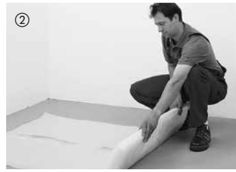
Always use 0.2 mm thick PE film overlapped by 30 cm as an underlay when laying your floor over floor screed. This should overlap in the 30 cm impact area. Extend underlay up all walls. After having installed the skirtings cut underlay at the upper edge of the skirtings.
