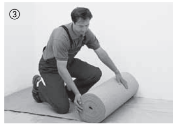
For sound insulation and to smooth out slight irregularities of the subfloor, unroll 2 mm thick cork underlay. Do not overlap. Our range of accessories also offers alternative insulation underlays. Asphalt-bitumen felt is not suitable for sound insulation. Do not use any additional insulation underlayment when laying laminate flooring with integrated insulation layer.
