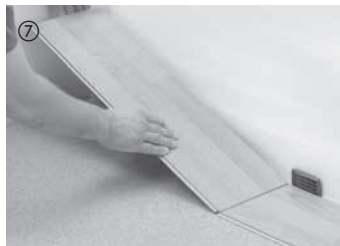
Cut the last board of the first row to size, leaving an expansion gap of 10–15 mm between the board and wall. Insert the board at a slight angle and rotate it down. The next row is started with the leftover piece of the first row (short side offset of at least 40 cm). This considerably reduces waste.
