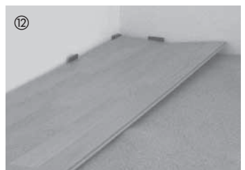
When you have interlocked the whole row on the long side and the short sides, you can lower it. Work from left to right.
