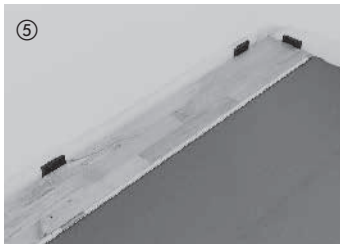
⑤ Starting in the right-hand corner of the room, align the boards of the first row with the tongue side parallel to the wall, and fix them in place with wall spacers or plastic spacers as you proceed (always keep an expansion gap of 10 - 15 mm (3/8" - 1/2") around perimeter).
