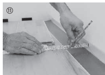
⑪ Cut to size and fit in the boards of the last row. Leave a gap of 10 to 15 mm between the boards and wall.
