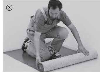
③ For sound insulation and to smooth out slight irregularities of the subfloor, unroll 2 mm thick luxury insulation layer. Our range of accessories also offers suitable insulation underlays. Asphalt-bitumen felt is not suitable for sound insulation. Parquet with integrated insulation layer is not suitable for glue-down installation.
