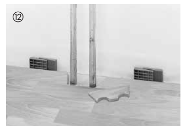
⑫ If radiator pipes protrude from the floor, drill or saw a cutout into the board (the size of the cutout depends on the radiator pipe and the required expansion space).
