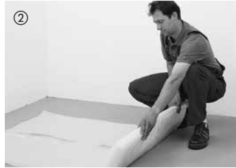
② Always use 0.2 mm thick PE film overlapped by 30 cm as an underlay when laying your floor over floor screed. This should overlap in the 30 cm impact area. Extend underlay up all walls. After having installed the skirtings cut underlay at the upper edge of the skirtings.
