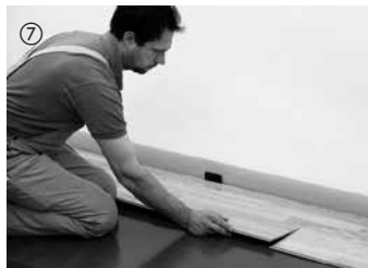
⑦ The next row is started with the leftover piece of the first row (short side offset of at least 50 cm). This considerably reduces waste. The rest of the installation is performed board-by-board. First, the boards are angled into the previous row along the long side by applying a small amount of force.
