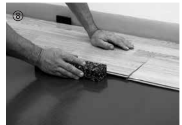
⑧ Tap edge gently with tapping block, if necessary.
