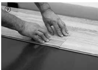
⑨ The board is then lowered in on the short side. Ensure here that the board is flush at the short side with the previously laid board. Pressure applied briefly to the side joint clicks in the board.
