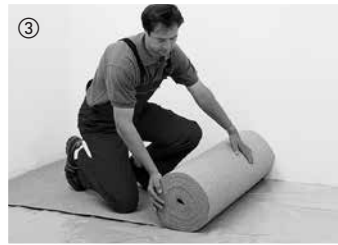
③ For sound insulation and to smooth out slight irregularities of the subfloor, unroll 2 mm thick cork underlay. Do not overlap. Our range of accessories also offers alternative insulation underlays. Asphalt-bitumen felt is not suitable for sound insulation. Do not use any additional insulation underlay when installing HARO Laminate Floor Silent Pro®.
