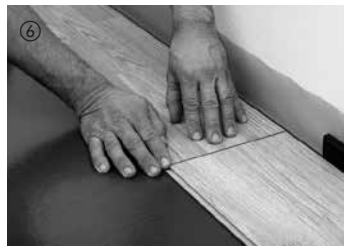
⑥ The remaining boards of the first row must be clicked in from above at the head ends into the previous boards. Pressure applied briefly to the side joint clicks in the board into the adjacent board. It is important to ensure that the first row is straight and exactly parallel to the wall. Cut the last board of the first row to size, leaving an expansion gap of 1015 mm (3/8" - 1/2") between the board and wall. Fit in the board and lay it flat.
