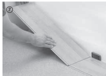
⑦ Cut the last board of the first row to size, leaving an expansion gap of 10–15 mm between the board and wall. Insert the board at a slight angle and rotate it down. The next row is started with the leftover piece of the first row (short side offset of at least 40 cm). This considerably reduces waste.
