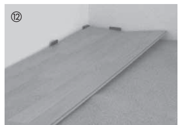
⑫ When you have interlocked the whole row on the long side and the short sides, you can lower it. Work from left to right.
