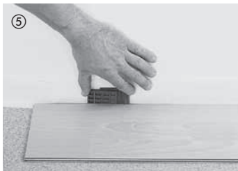
⑤ Starting in the right-hand corner of the room, align the boards of the first row with the tongue side parallel to the wall, and fix them in place with wall spacers as you proceed (always keep an expansion gap of 10–15 mm (3/8"–1/2") around perimeter).
