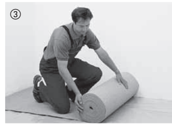
③ For sound insulation and to smooth out slight irregularities of the subfloor, unroll 2 mm thick cork underlay. Do not overlap. Our range of accessories also offers alternative insulation underlays. Asphalt-bitumen felt is not suitable for sound insulation. Do not use any additional insulation underlay when installing HARO Laminate Floor Silent Pro®.
