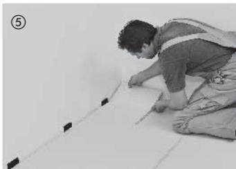
Cut the last board of the first row to size, leaving an expansion gap of 1015 mm (3/8" - 1/2") between the board and wall. Fit in the board and lay it flat. The next row is started with the leftover piece of the first row (short side offset of at least 18 cm). This considerably reduces waste.
