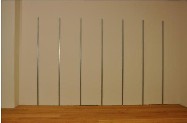
3. Attach the fastening rails to the wall at a distance of 50 cm (see Item 1) using appropriate wall plugs and screws. Slight wall irregularities can be levelled out using spacers or wooden wedges.
