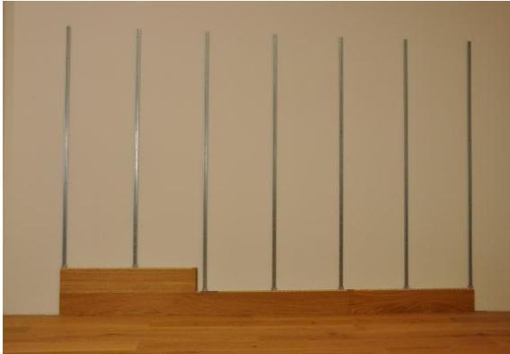
13. Start the second row with the leftover piece from the first row. The remaining installation is performed board by board from left to right.
