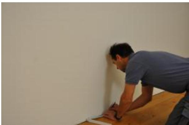
1. Measure the distances and the height of the fastening rails and draw these on the wall in accordance with the required wall panelling area. (Rail distances with HARO Parquet Series 4000 approx. 50 cm.)
