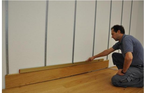
4. Parquet boards are installed from left to right. The tongue side points towards the floor.
