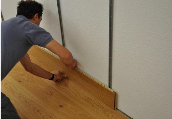
7. When the initial clips are attached, the boards are simply clicked into the fastening rails.
