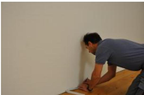
1. Measure the distances and the height of the fastening rails and draw these on the wall in accordance with the required wall panelling area. (Rail distances with HARO Tritty 100 Laminate approx. 50 cm.)
