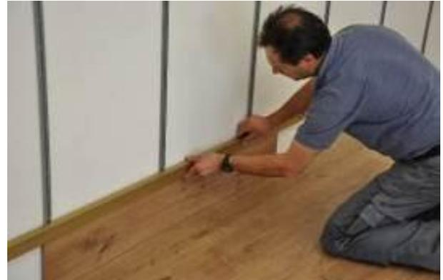
4. Laminate boards are installed from left to right. The tongue side points towards the floor.
