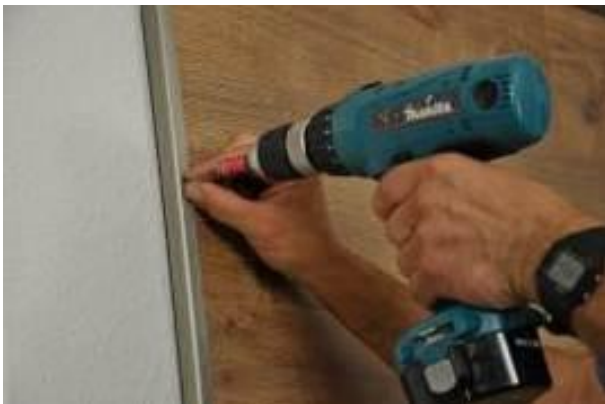
18. Attach the aluminium cover moulding
