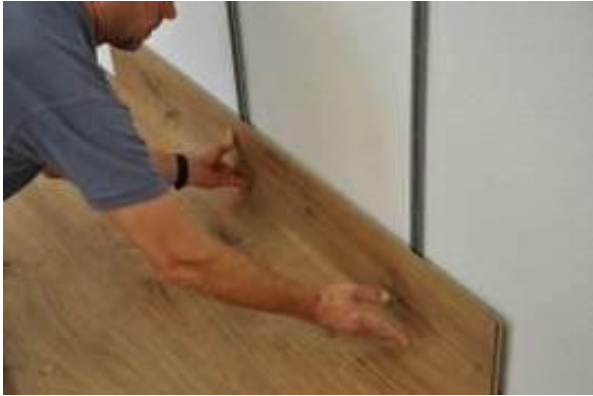
7. When the initial clips are attached, the boards are simply clicked into the fastening rails.
