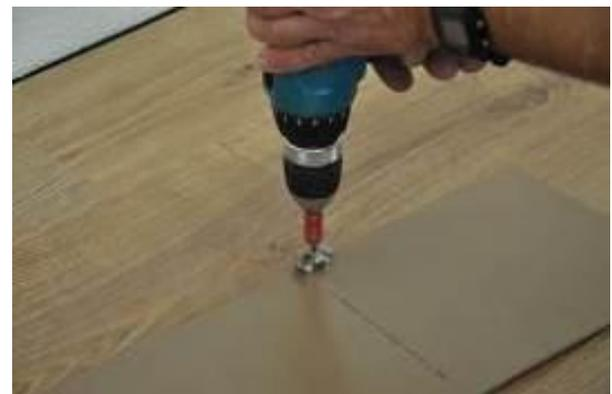
6. Use the enclosed screws to attach the initial and end clips (at external span of approx. 2 cm). Tighten the screws but not excessively.
