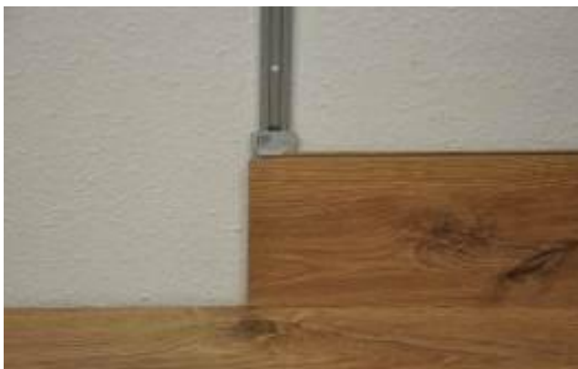
11. Secured fastening clip Use the laminate floor fastening clips for the remaining installation in order to secure the boards on the groove side. The clip is simply screwed into the fastening rail and pushed down into the groove.
