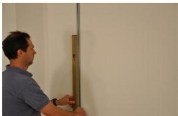
2. Make sure the rails are perpendicular and draw in the drilled holes (include a drilled hole approx. every 60-70 cm). Use a standard hacksaw to cut the fastening rail to the desired length.
