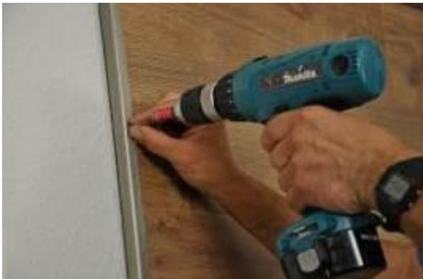
18. Attach the aluminium cover moulding
