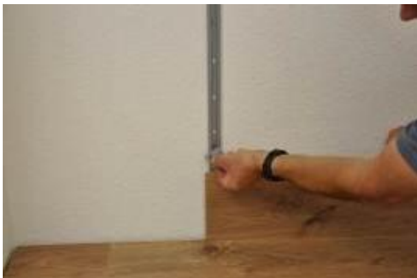
9. Attach the fastening clip from above.
