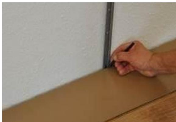
5. Use the initial and end clips to install the boards of the first row. In preparation mark the respective centre of the rail on the rear of the board.
