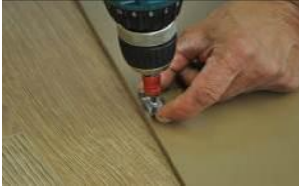
16. Attach the end clips.
