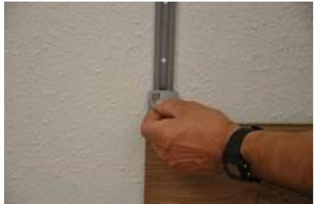
10. Push the fastening clip down into the connection.
