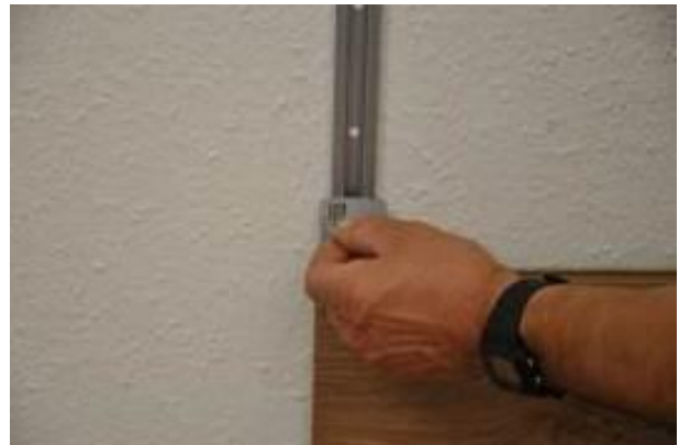
10. Push the fastening clip down into the connection.
