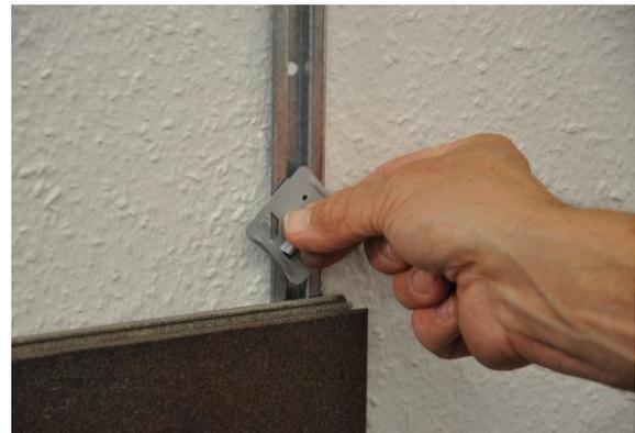
9. Use the Celenio fastening clips for the remaining installation in order to secure the boards on the groove side.
