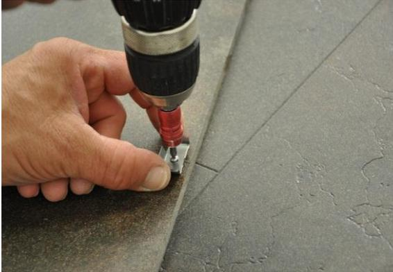
6. Use the enclosed screws to attach the initial and end clips (at external span of approx. 2 cm). Tighten the screws but not excessively.
