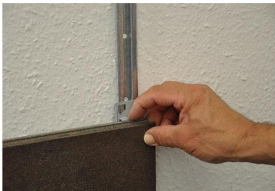
10. The clip is simply screwed into the fastening rail here.
