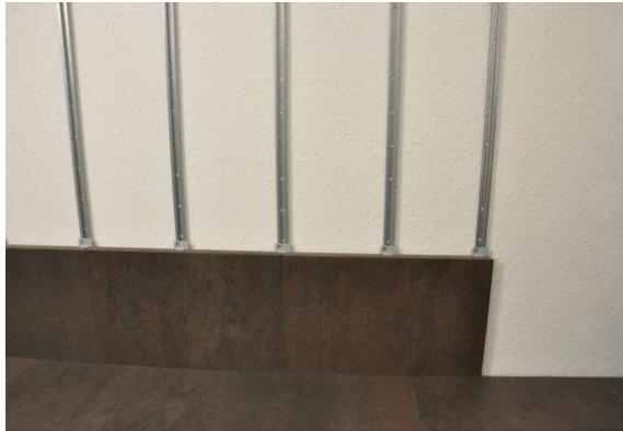
12. Attach the fastening clips to each fastening rail.
