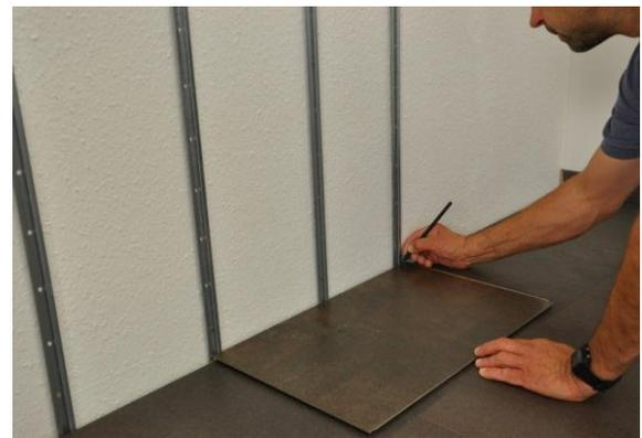
5. Use the initial and end clips to install the boards of the first row. In preparation mark the respective centre of the rail on the rear of the Celenio board. Note that initial and end clips are required with the outermost boards of the first row.
