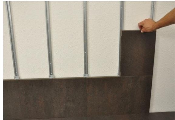
13. The next row is started with the leftover piece (half the board width) of the first row (short side offset = half board length). The remaining installation is performed board by board from right to left.
