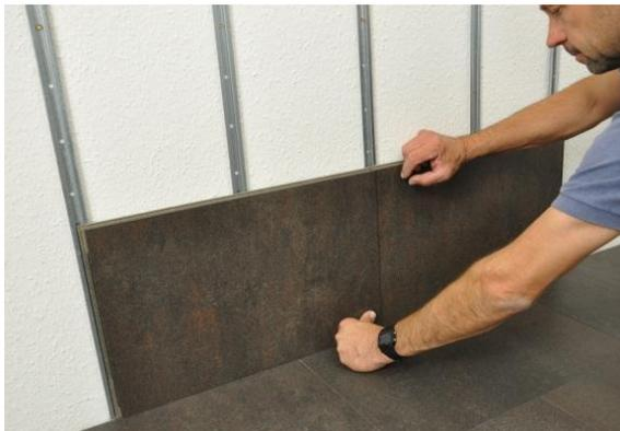
8. Install the first row from right to left and lock the individual boards to the edge joints.
