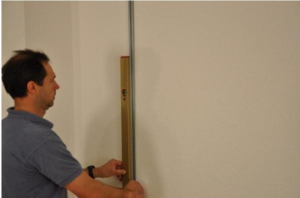
2. Make sure the rails are perpendicular and draw in the drilled holes (include a drilled hole approx. every 60-70 cm).
