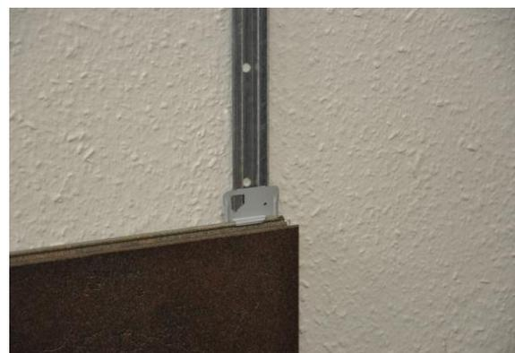
11. The clip is then pushed down into the groove.
