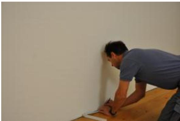
1. Measure the distances and the height of the fastening rails and draw these on the wall in accordance with the required wall panelling area. (Rail distances for Celenio 8x350x526 mm: 35 cm – measured from the centre of the rail.)
