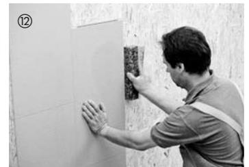
If necessary the row can be straightened using a tapping block. This also ensures a perfect joint flush, among other factors.
