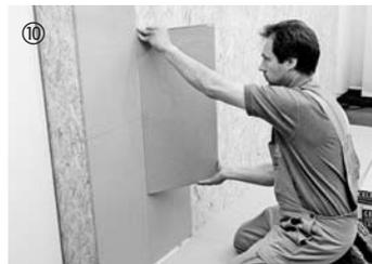
The second board of the second row must first be angled in on the long side and then clicked in on the head ends from above into previous boards. Ensure here that the board adjoins at the short side with the previously laid board. Pressure applied briefly to the side joint clicks in the board.
