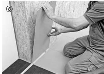
Beginning on the bottom left wall, the first board is placed so that the groove long side is on the right-hand side. If the boards are laid in cross format, the groove long side must point up. Expansion space to the floor or room corners: at least 5 mm. In the following pictures the boards are laid in high format.
