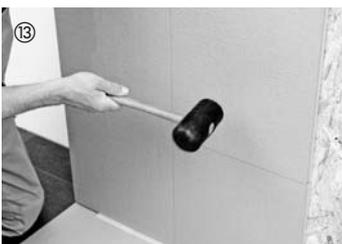
The CELENIO boards are fixed using a rubber mallet and therefore guarantee adequate adhesive transfer with the glue.
