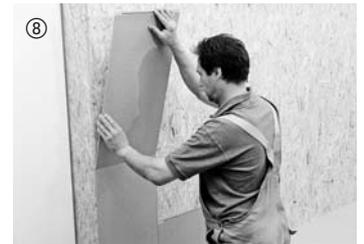
After applying the glue, the second board of the first row must first be clicked on the short side into the first board, lowered and pressed on.
