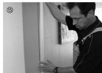
After installation and as required, fix outer and inner corners to the wall – you're done!
