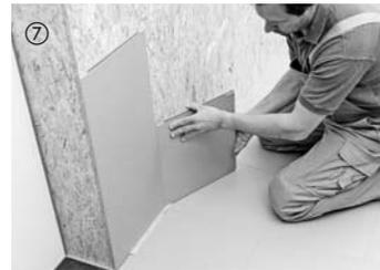
The next cut-to-size board is only angled into the long side of the first board and pressed on after applying the glue in half-board staggering.
