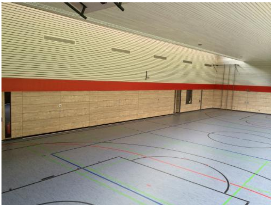
...and around 150 sq. m. tailor-made HARO Sports protective walls Protect Classic in Pinie Tessin pattern design were installed.
