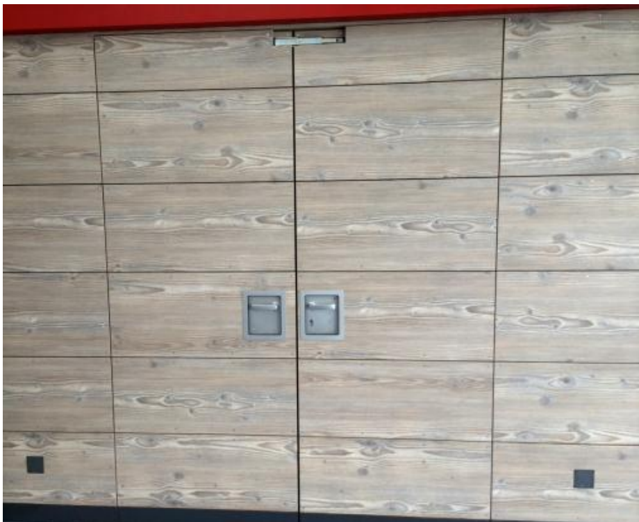
...as well as a double-leaf entrance door make the renovation perfect
